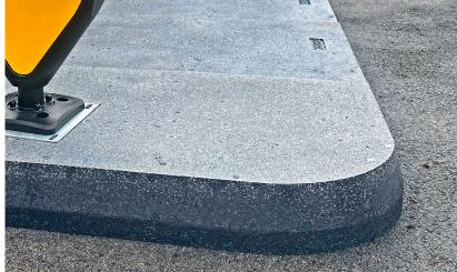
"Construction of a traditional pre cast concrete kerbed island on Waterloo Road would have resulted in a road closure over several days due to the narrow configuration of the carriageway. A bespoke surface-mounted solution from Rosehill Highways was installed in a just one and a half hours under minimal traffic management with the road opened back up to all traffic flows immediately after the installation."
